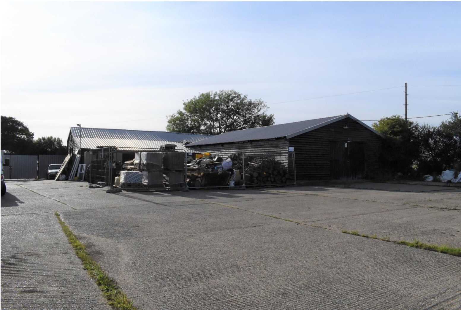
Plate 7: View across the PDA from the entrance gate (facing NW).
